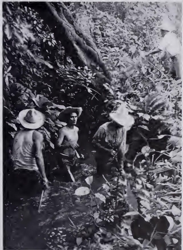
DITCH DIGGING IN MEXICO
